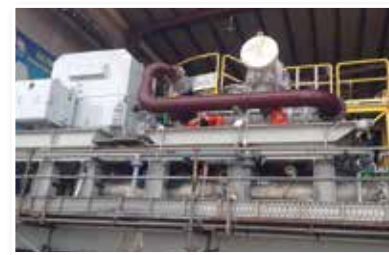
Gas chiller - Africa offshore 4032XLLL / 2400kW
